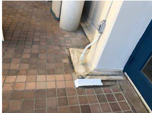
Photo #4: Non-asbestos containing quarry tiles system including tile, grout and mortar substrate.
