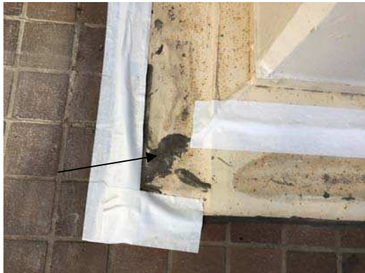
Photo #6: Non-asbestos containing caulking at the metal flashing.
