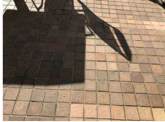
Photo #2: Non-asbestos containing quarry tiles system including tile, grout and mortar substrate.
