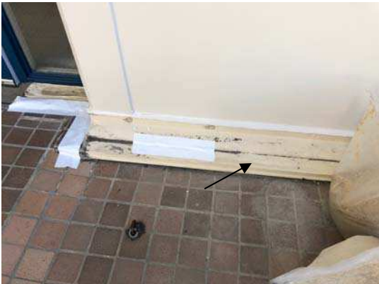
Photo #5: Lead containing beige paint on the metal flashing.
