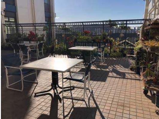
Photo #1: Existing sundeck.
