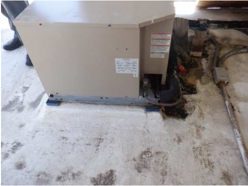
Photo 7: Asbestos-containing black tar/silver paint on the roof pad and pipe penetration sealant.
