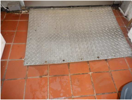
Photo 1: Non asbestos-containing red quarry floor tile and grout/ mortar adjacent to the freezer.
