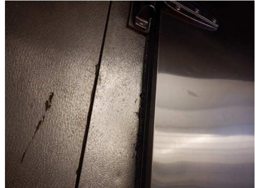
Photo 4: Non asbestos-containing gray caulking on freezer joint sealant.
