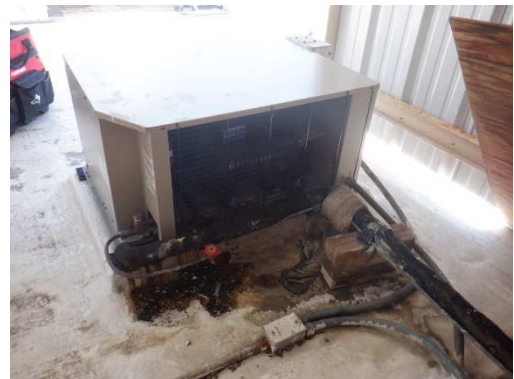
Photo 6: Non asbestos-containing black foam and adhesive pipe insulation connecting the condensing unit.
