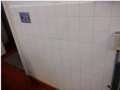
Photo 5: Asbestos-containing mortar behind to the non asbestos-containing glazed white ceramic wall tile and grout adjacent to the walk-in freezer. Non lead-based glazed white ceramic coating.
