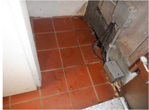
Photo 8: Kitchen red quarry floor tile. Non lead-based glazed red coating.
