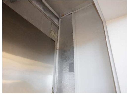
Photo 2: Non asbestos-containing silver foil/paper cover and red fiberglass wall insulation adjacent to the freezer.
