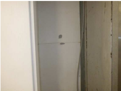
Photo 9: Plaster wall adjacent to the freezer. Non lead-based beige paint.
